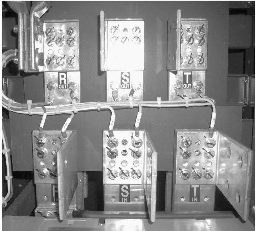
Figure 6 - Automatic Bypass Switchboard Terminations and Conduit Landing Areas
