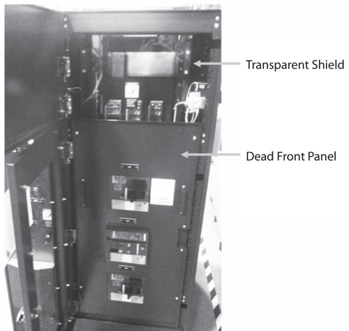
Figure 5 - Main Power Terminals (front view)
