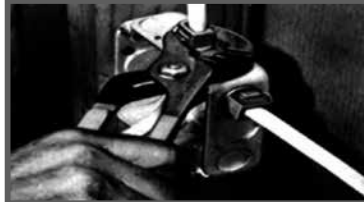
Press locking wedge into cavity that locks onto cable.
