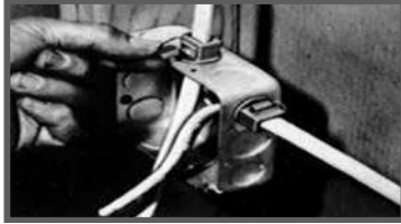
Snap captive locking wedge into connector's cavity.
