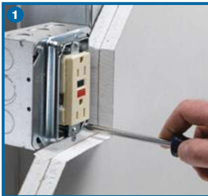
Loosen... The two adjustment screws located on opposing corners of the mud ring.
