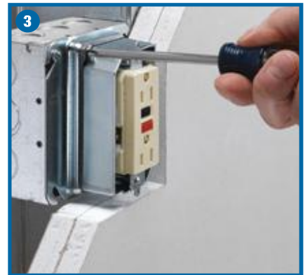
Re-tighten... Adjustment screws.
