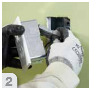
2 Connect the wiring device.
