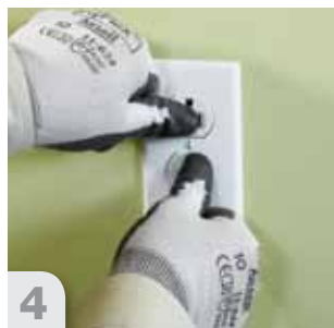
4 Push the device assembly— and you're done!
