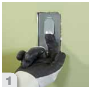
1 Remove the protective plate.
