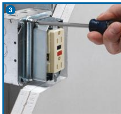
Re-tighten... Adjustment screws.
